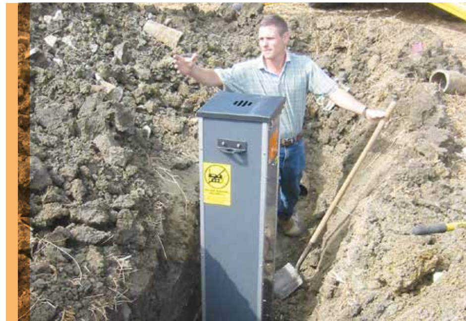
^ Installation of a drainage water control structure in a drain tile.
