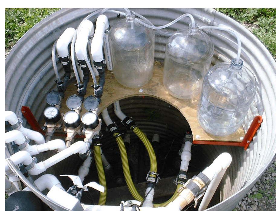
Fig. 1. Continuous subsurface drain flow measurements and composite water sampling.
